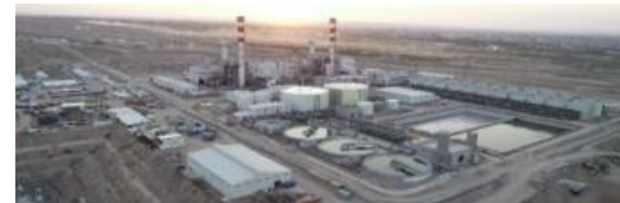
Turakurgan Thermal Power Station Japan International Cooperation Agency
